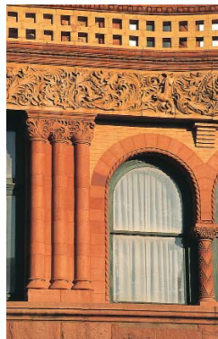
A thorough cross-referenced index is helpful in locating desired details outside their categories, such as this arched window and frieze detail found in a photograph in the "Pilasters & Engaged Columns" section.
