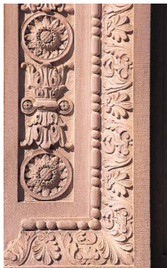
The author provides detailed, technical captions: "Corner detail of enriched ovolo molding with trailing foliated pattern; bead-and-reel framing foliated design flanked by rosettes."
